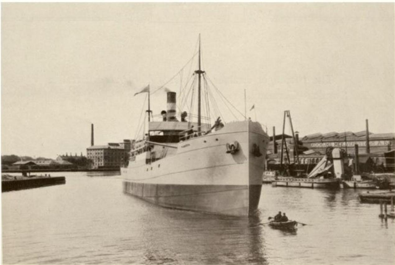
Kockums: "The illustration shows one of the steam-cargo-ships of 2200 tons d. w., built by us. This ship is equipped with Triple-Expansion Engines 800 I.H.P. of our own make."
